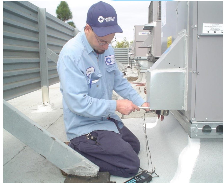
OSA inlet with a barometric damper
